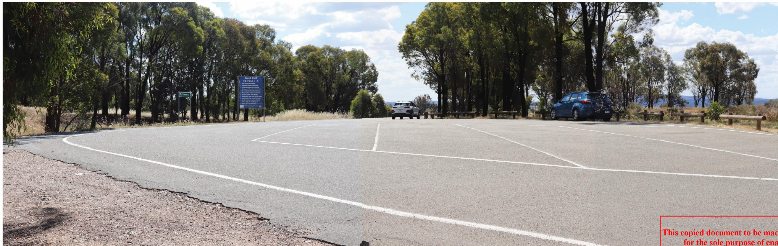
Image: VPL 02 – Mokoan Rest Area Southbound car park, view north west
