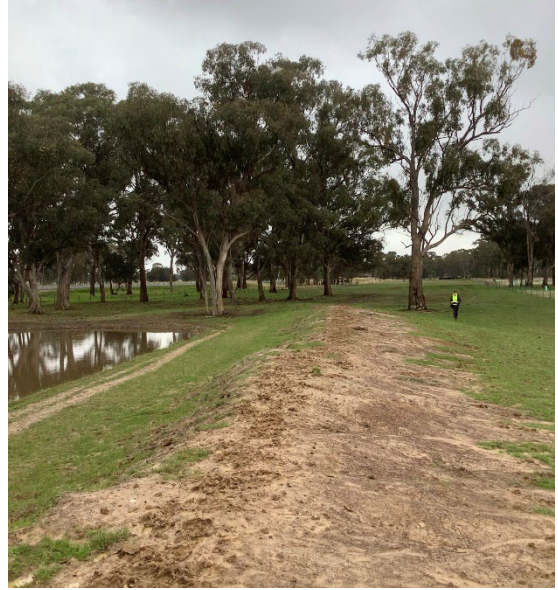
Photo 4.6 Bunded wall of farm dam
